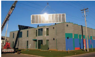
Solar panels are set in place
