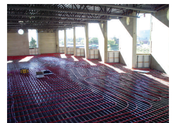
Radiant floor heating installation
